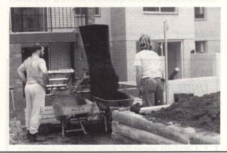
it to carry a range of materials including sand, woodchips, bricks, blocks, tiles, gyprock, small concrete pours and rubble. Furniture and cartons can also be lifted or lowered.
