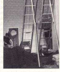
Ladder Lift can be carried by one person and erected in areas where space is limited.
